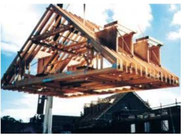
Above left: An example of ground level erection of "RiR" trussed rafters. Above right: A typical "Room in the Roof" installation.
